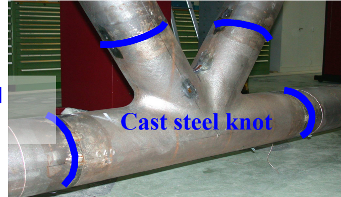
Conventional butt welds
